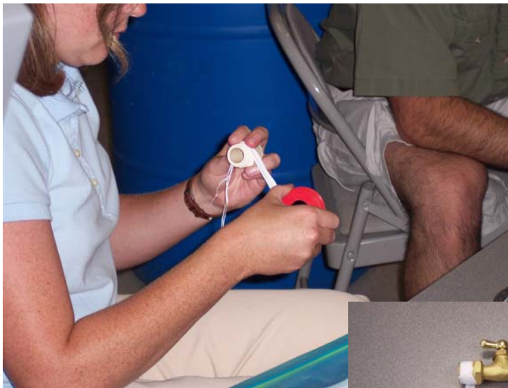
Wrapping tape around the hose spigot
