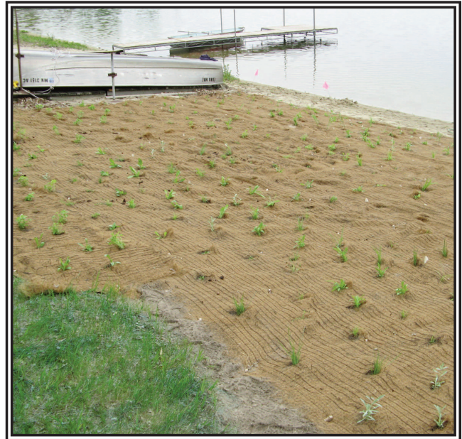
One of the six lots on Spirit Lake, showing plants in an erosion control blanket that will help retain moisture in the sand. Photo credit: Karen Terry
