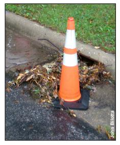
Stormwater runoff from curbs and gutters along streets carry sediment, debris, and other pollutants directly to storm sewers. Frequently, urban stormwater flows untreated to receiving waters.
