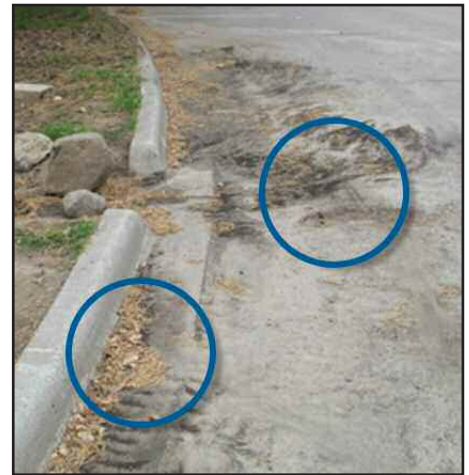
Sediment and debris, such as the sand and dead vegetation in this photo, should be removed before they enter the rain garden.
