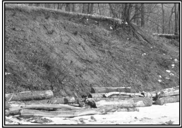
Logs for shoreline stabilization
