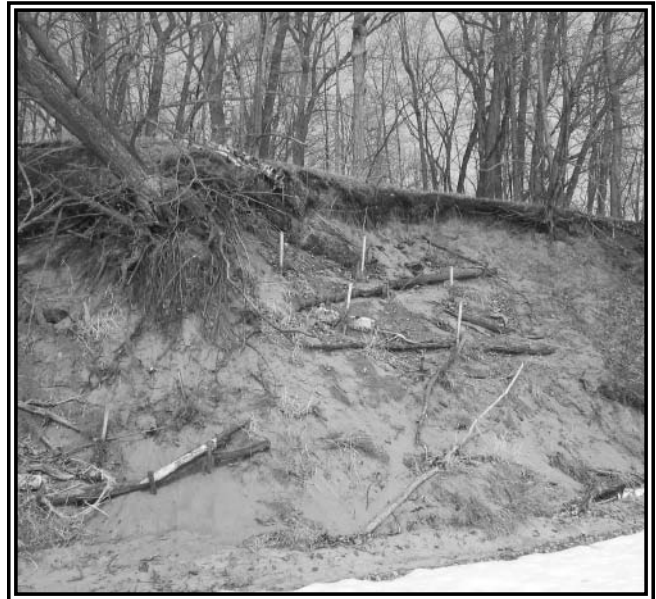
County Island before erosion control
