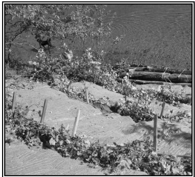
Erosion control in place
