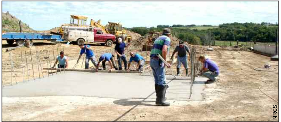
Constructing pads for structures to prevent manure from running off site.
